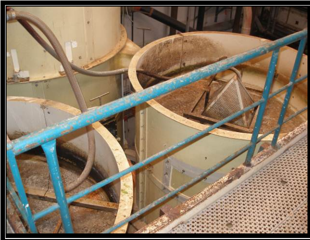
Figure 7. Fluidised bed biofilters at Jupiter Eel, Stege, Denmark.
