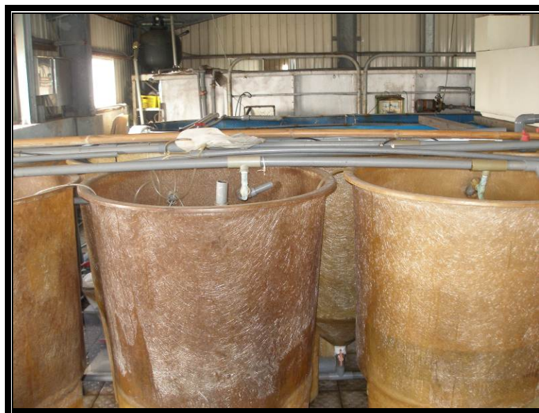
Figure 11. Egg incubation and larval rearing tanks at the Freshwater Aquaculture Research Centre, La Kung
